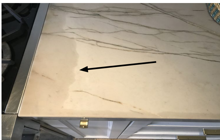
Intrusion of oil from the side. Oil collecting between the cook top and countertop gradually seeps into the stone.
