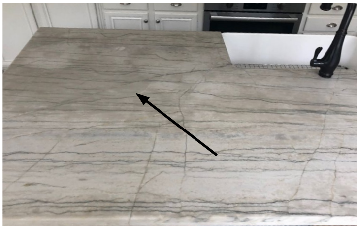
Intrusion of oil in Kitchen Island.
