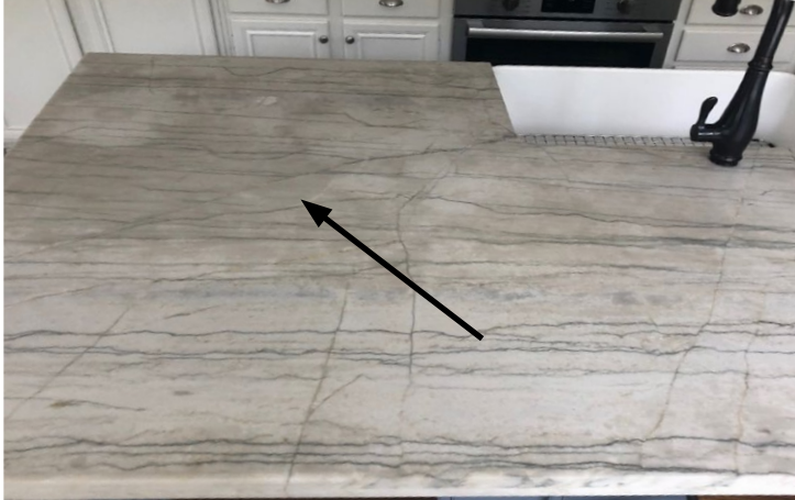
Intrusion of oil in Kitchen Island.
