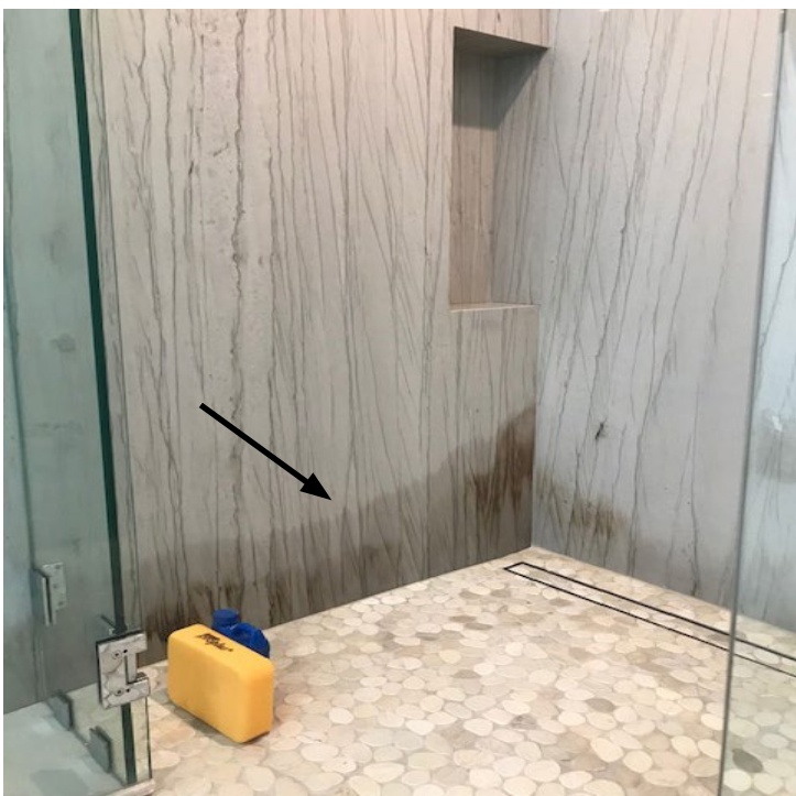
Water intrusion in a shower. Sealing front and back of quartzite is very important.
